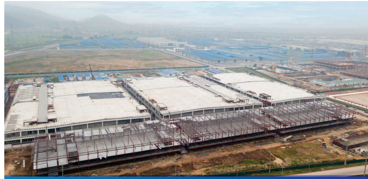
FUKANG TECHNOLOGY FACTORY
