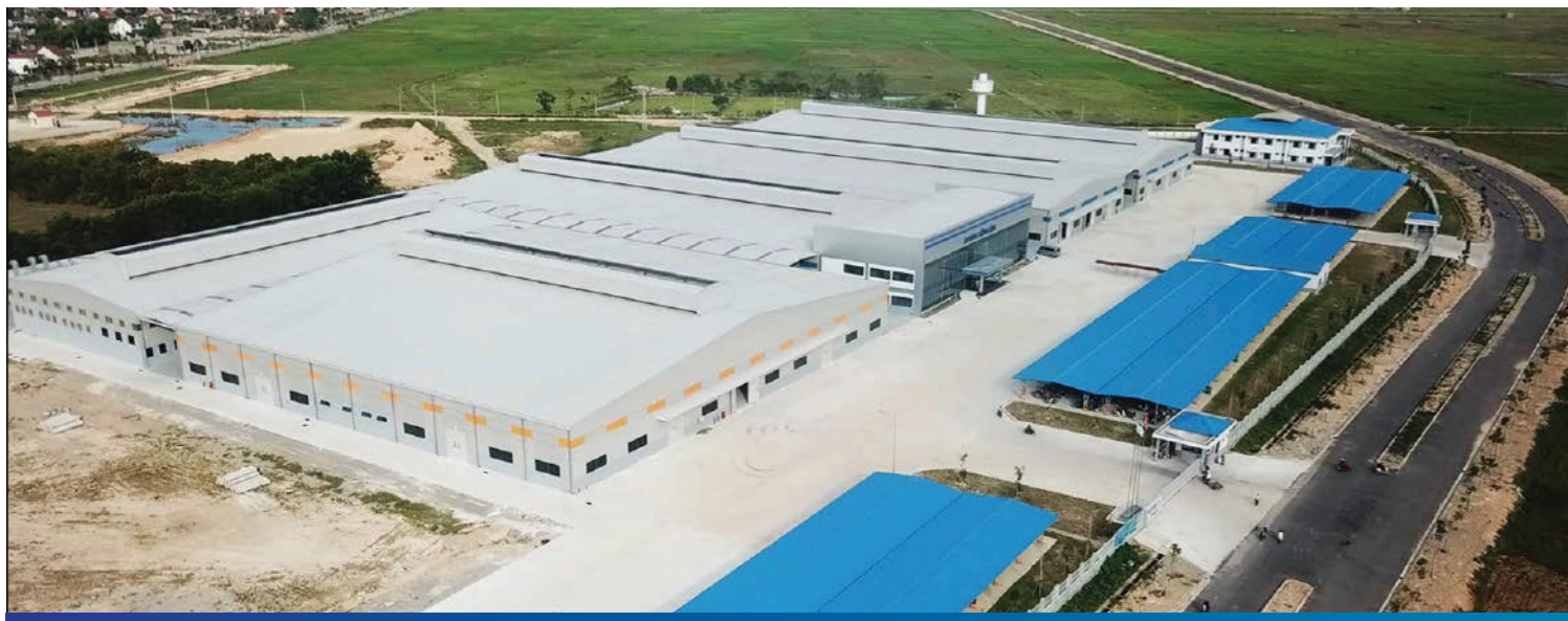
HAIVINA HONG LINH FACTORY
